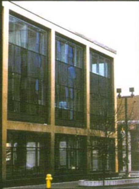
PROJECT: Government of Canada Building SUBMITTED BY: Centis Tile & Terrazzo Inc.
