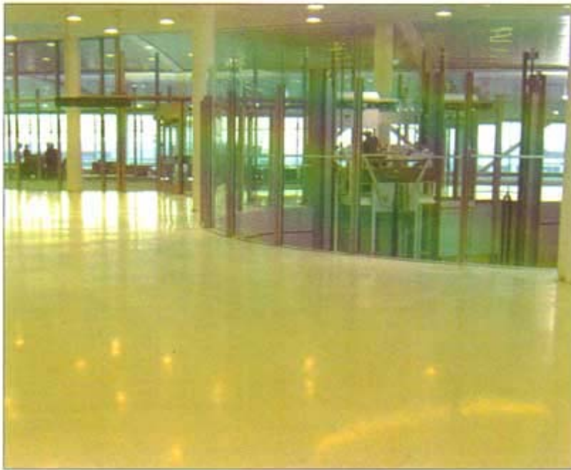
Terrazzo Installation, Rotunda Area
