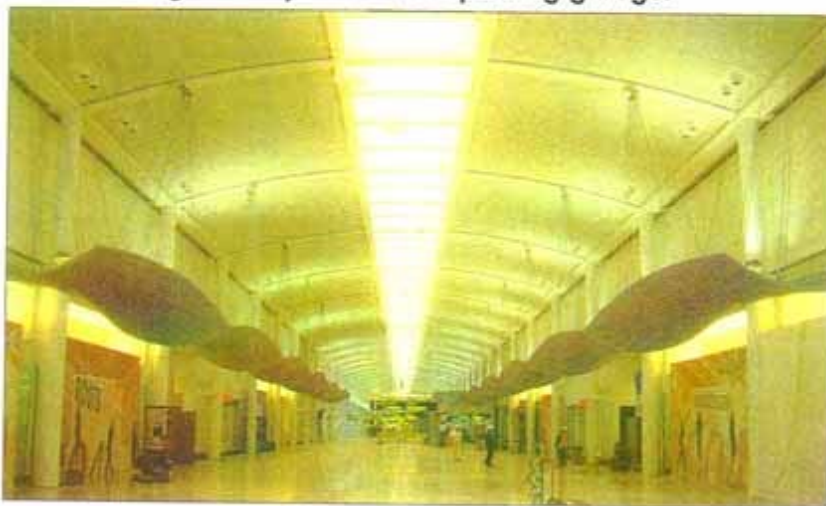
Pier E, Hammerhead on Level 2 of Terminal One. 90% of the granite was honed and 10% was flamed on the TMT/GEM project Courtesy of PCL/AECON
